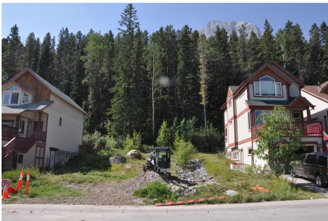
Photo 4-3. Photograph along Wilson Way looking upstream. One lot was left unoccupied to allow water flow in the riprapped channel which then enters a culvert below Wilson Way. BGC photograph of July 25, 2013.
